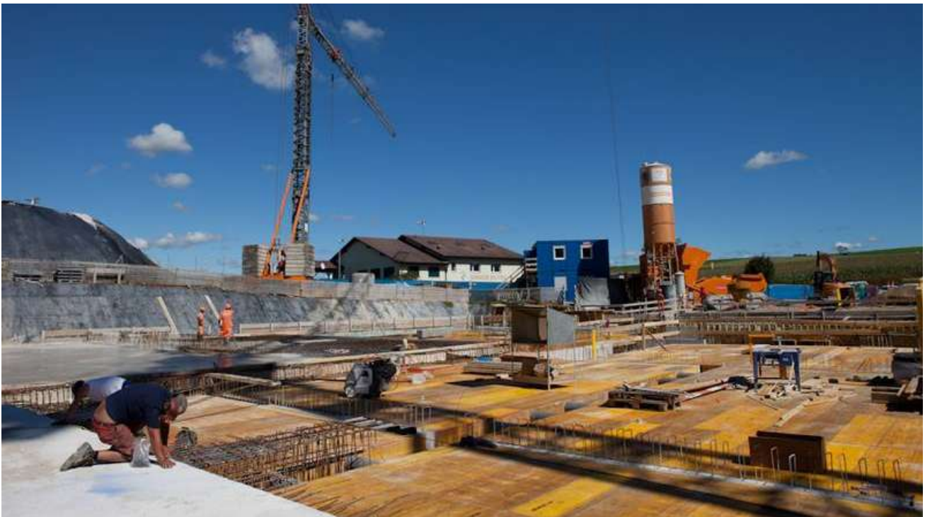
New Research and Archiving Centre, under construction in Penthaz (February 2011)
