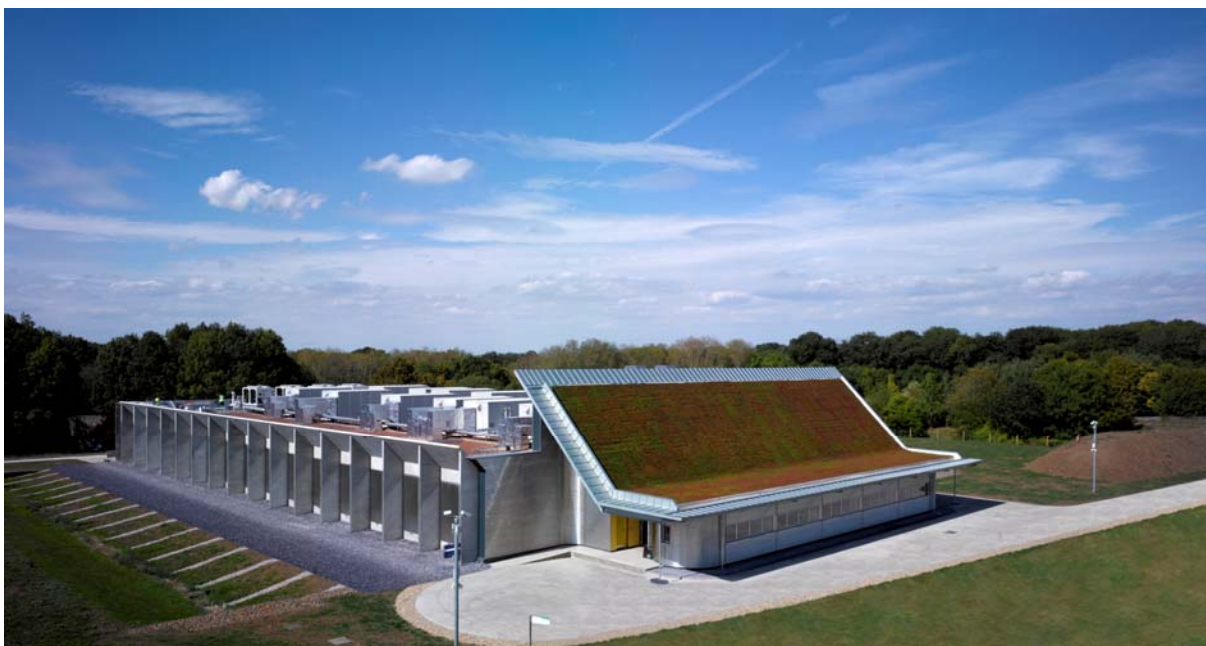
The new BFI film storage facility at Gaydon
