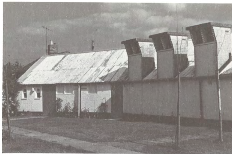
Existing structures are sometimes adapted to film storage. Here, nitrate vaults have been constructed inside some old farm buildings.
