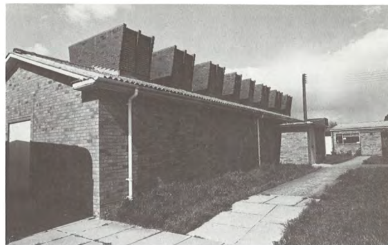
Modern nitrate storage vaults. The large blowout vents are required to release gas and avoid explosion in case of a fire.
